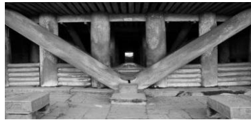
Figure 14: Ehomo dan ndriwa (connecting and buffering poles)
