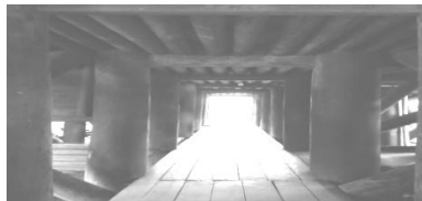
Figure 15: Arö mbatö (basement or floor under traditional house)
